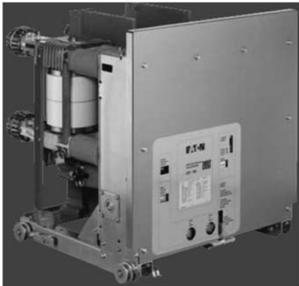
VCP-WG Breaker (Front View)
