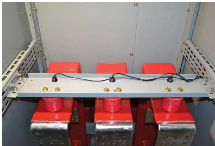
Figure 5.1-10. Typical Install for Continuous Thermal Monitoring Sensors
